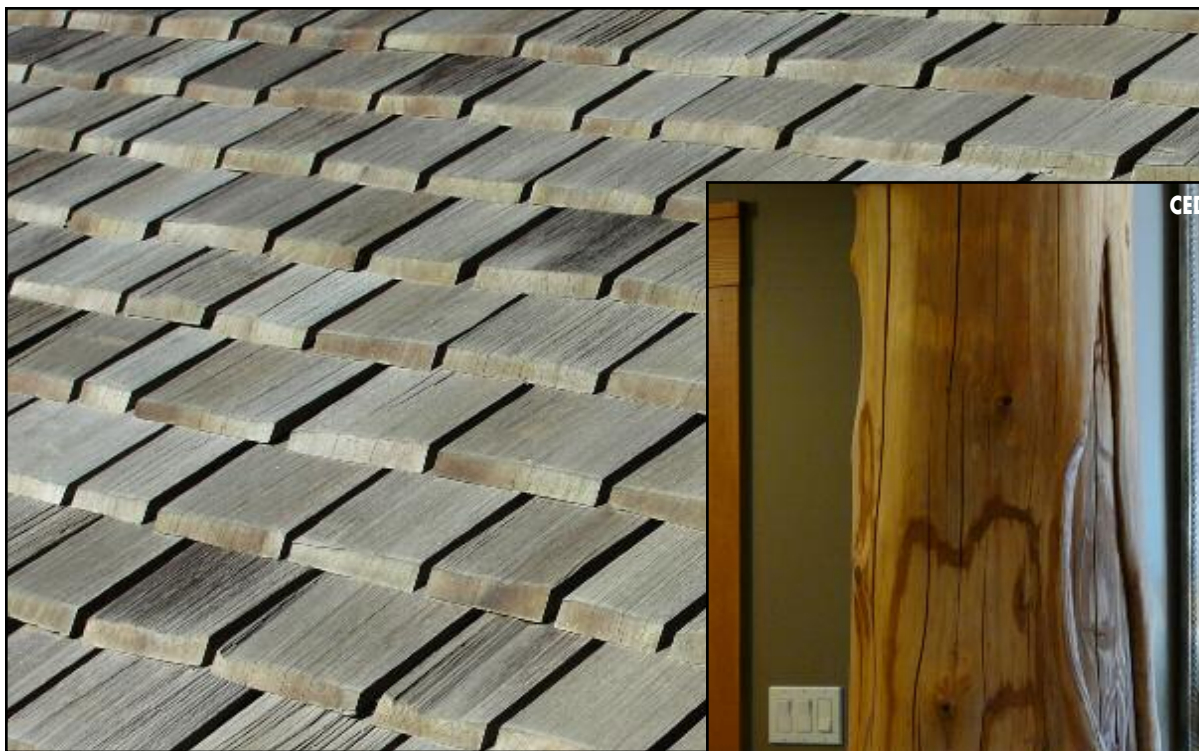
1 INCH THICK WESTERN RED CEDAR SHAKES WITH BEVELED BUTTS WERE USED ON THE ROOF.
